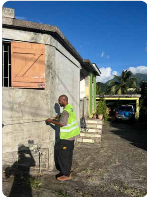
Housing pilot assessment, Dominica. Photo credit: @Build Change
