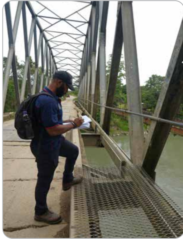
Bridge assessment, Papua New Guinea. Photo credit: @GGGI
