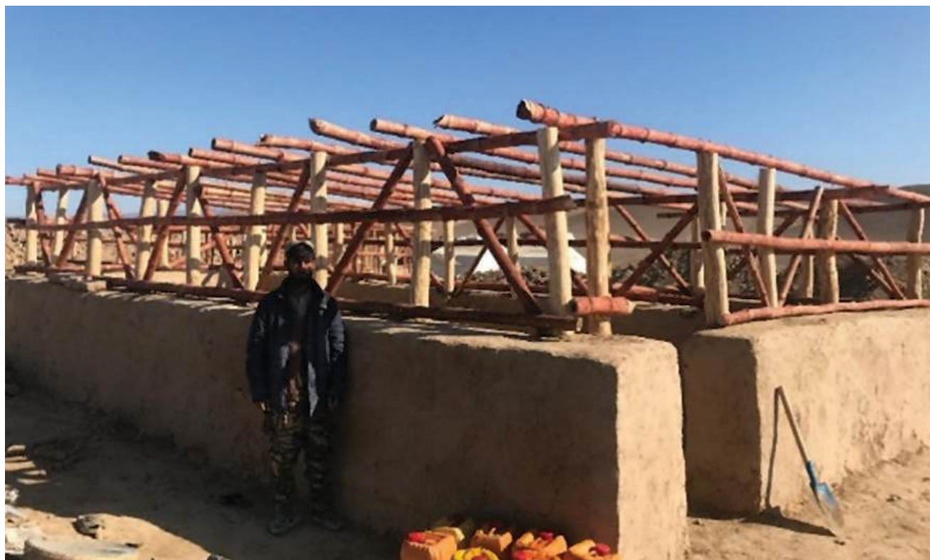
Image 4: Structure of transitional shelters, Chahak village, Herat
