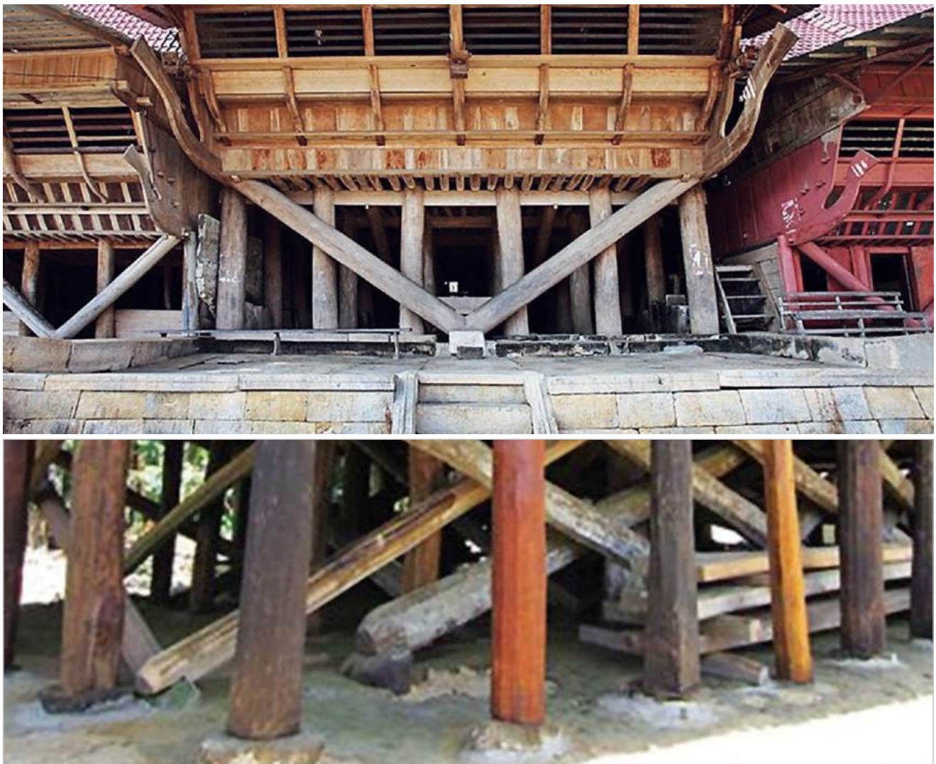
Image 5: Omo Hada disaster-resilient components: (top) elevated design (reduces humidity and prevents flooding) and driwa (V-shaped supports installed diagonally between vertical posts under the house); (middle) stone pedestals (can shift with horizontal forces without breaking during earthquakes); (bottom) high roofs made of sago palm (reduce heat radiation)
