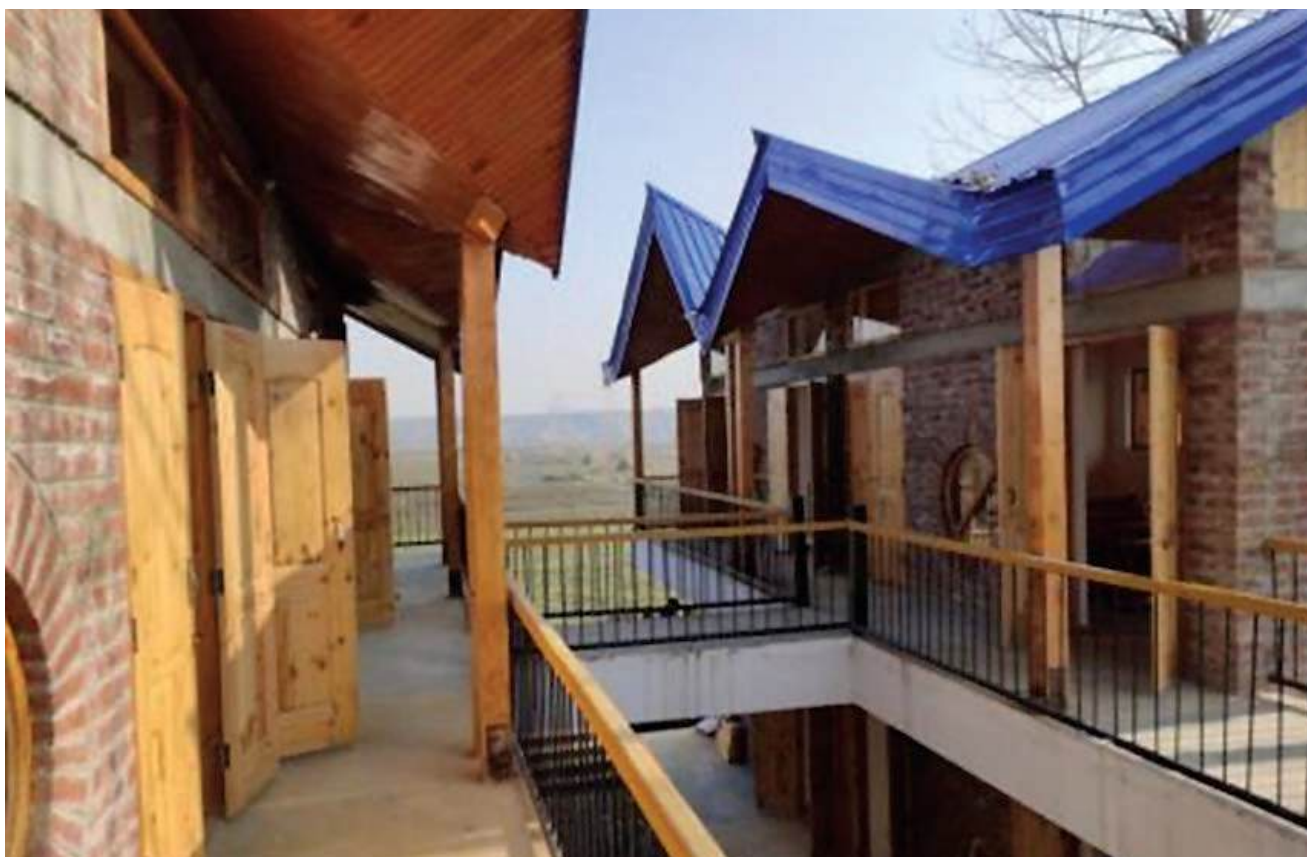
Image 4: First-floor corridor of Bajibagh School, featuring locally crafted wooden joinery, sloped metal roofing, and child-friendly design elements for safety and climate adaptation
