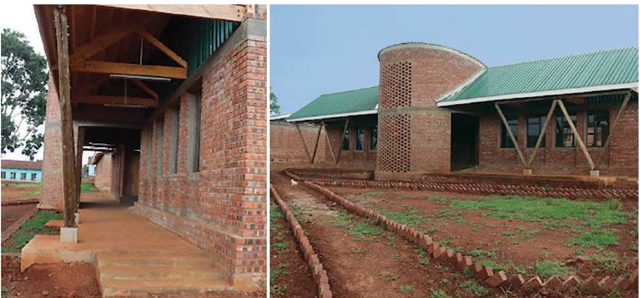
Image 4: Double truss timber roof system with V-shaped timber post supports
