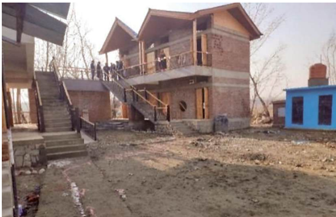
Image 2: Flood- and earthquake-resilient school building at Govt. Girls Middle School, Drangbal, showcasing community-led reconstruction and GRIHA-compliant design, seismic gap, load bearing structure, gable ends reinforced
