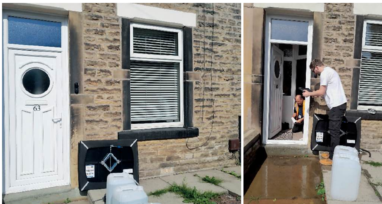
Image 3: Property benefiting from a 'stable' style flood resilient door to create an escape route to evacuate the property without compromising its flood resilience
