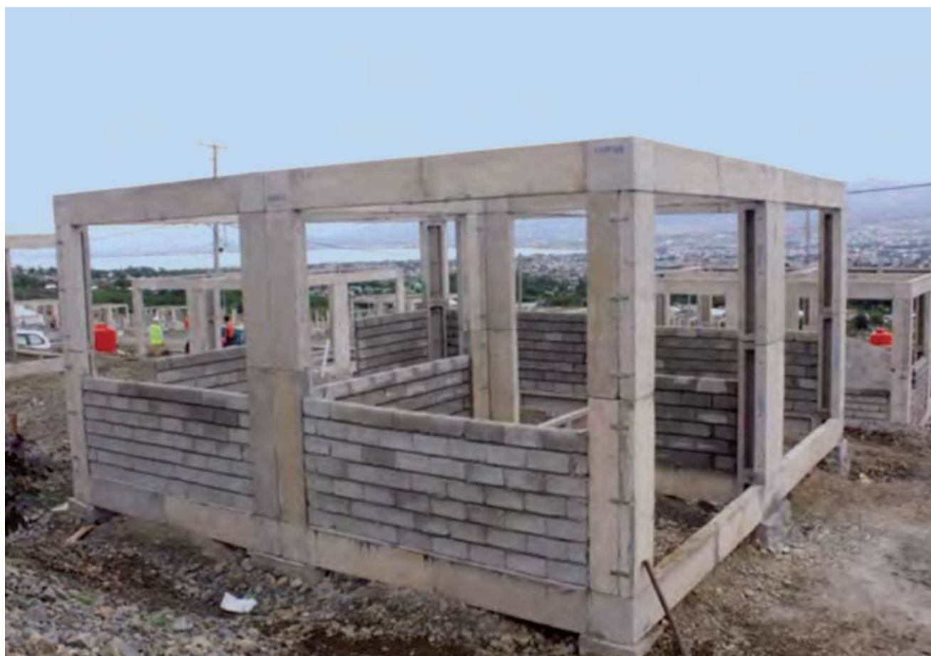
Image 1: The RISHA-type permanent housing built in Duyu, Palu, Central Sulawesi, during the construction process
