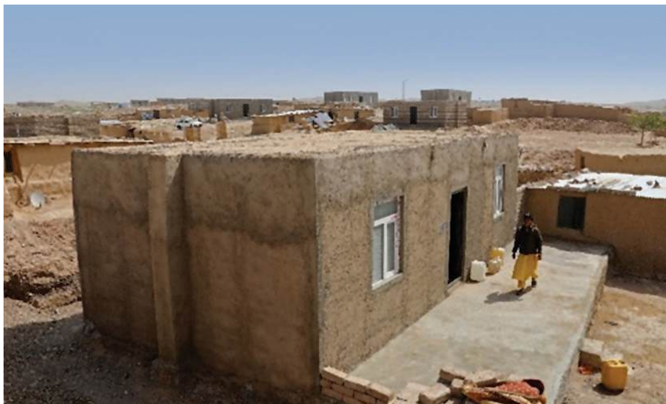
Image 6: Durable shelters constructed in Chahak village, using CSEBs and incorporating seismic features
