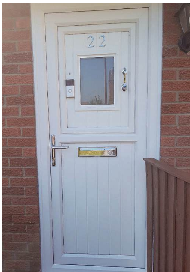
Image 3: Property benefiting from a 'stable' style flood resilient door to create an escape route to evacuate the property without compromising its flood resilience
