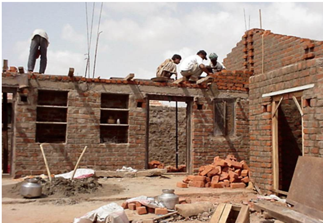
Image 2: Brick masonry building with reinforced cement concrete seismic bands
