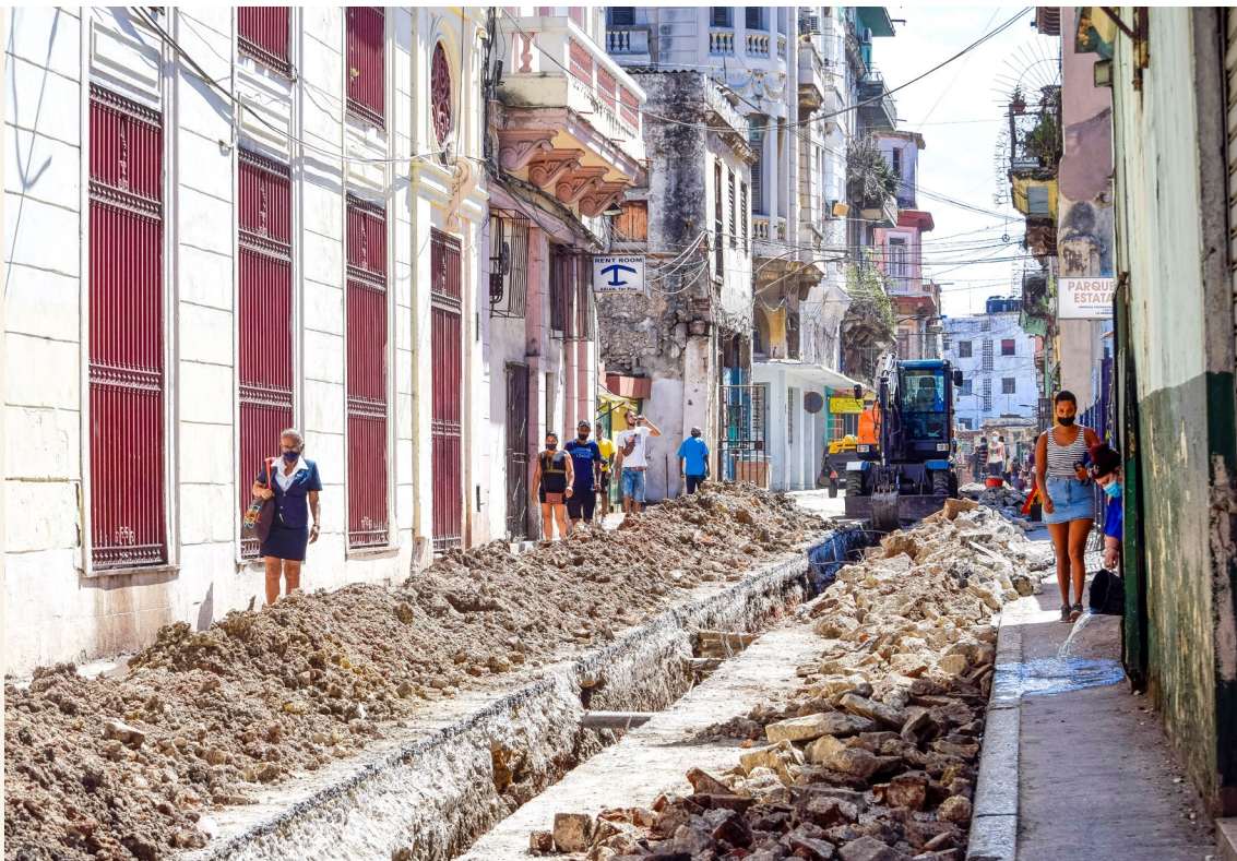
Construction and installation of new water pipes in Havana, Cuba Source: iStock
