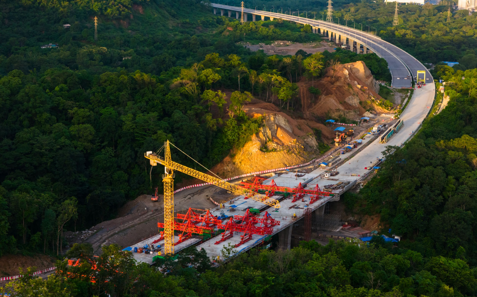
Highway bridge construction in Thailand Source: Getty Images
