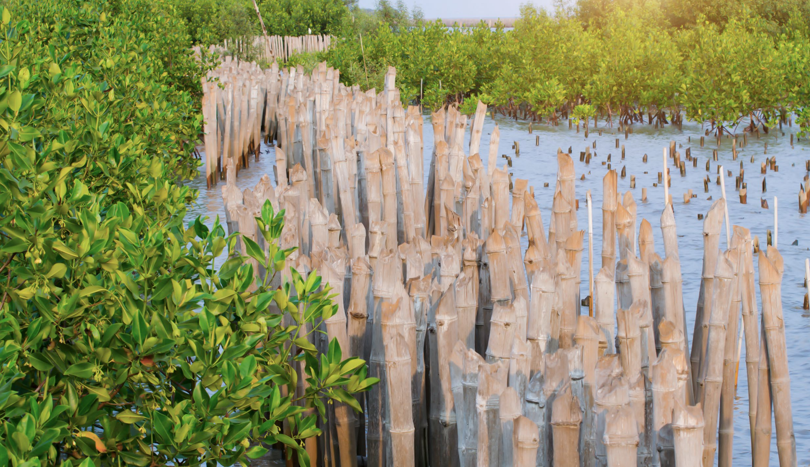
A bamboo fence in Indonesia helps protect from water erosion Source: Getty Images
