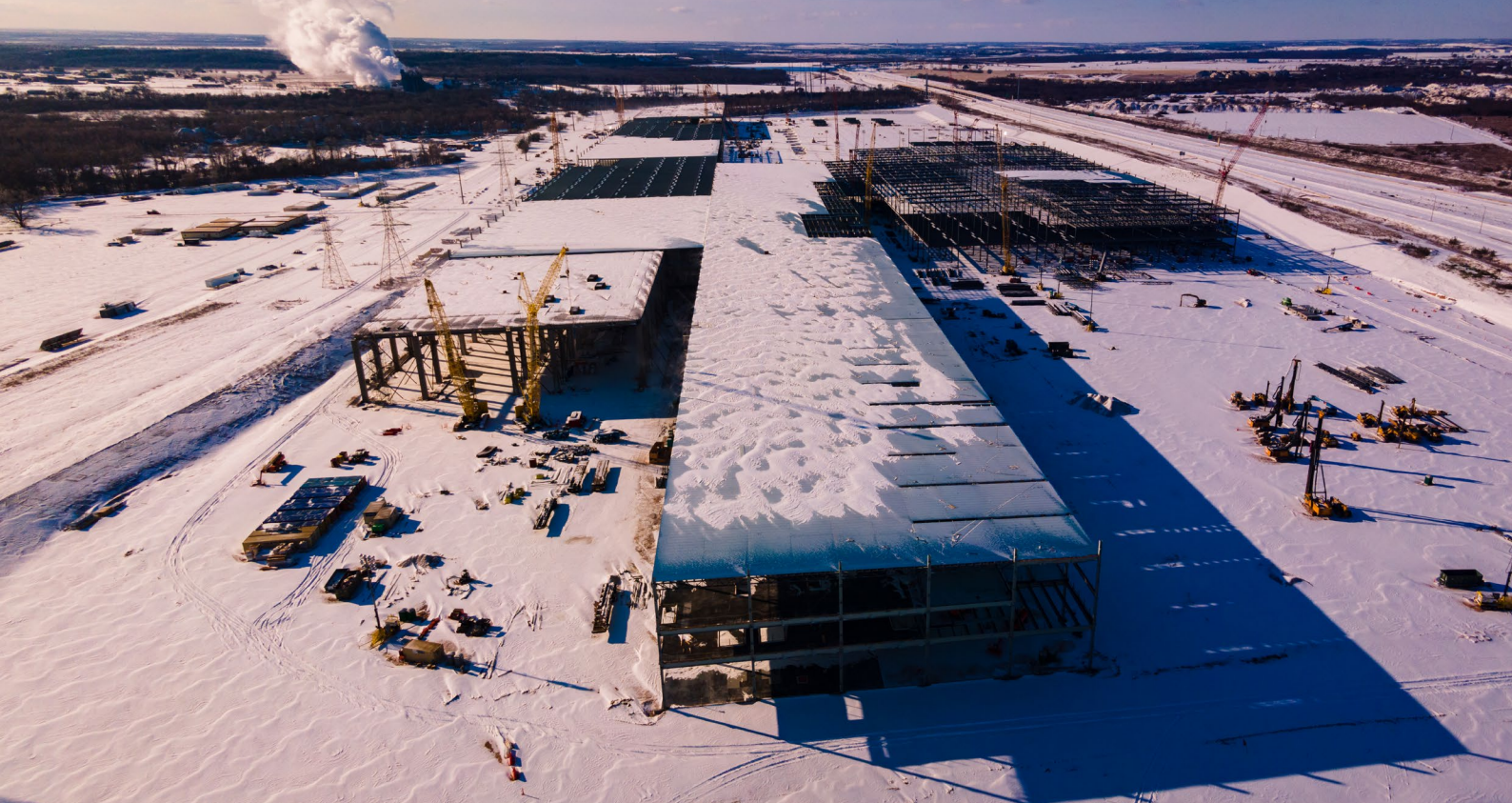
Winter Storm Uri covered the Tesla Giga Texas facility outside in Austin Source: Shutterstock
