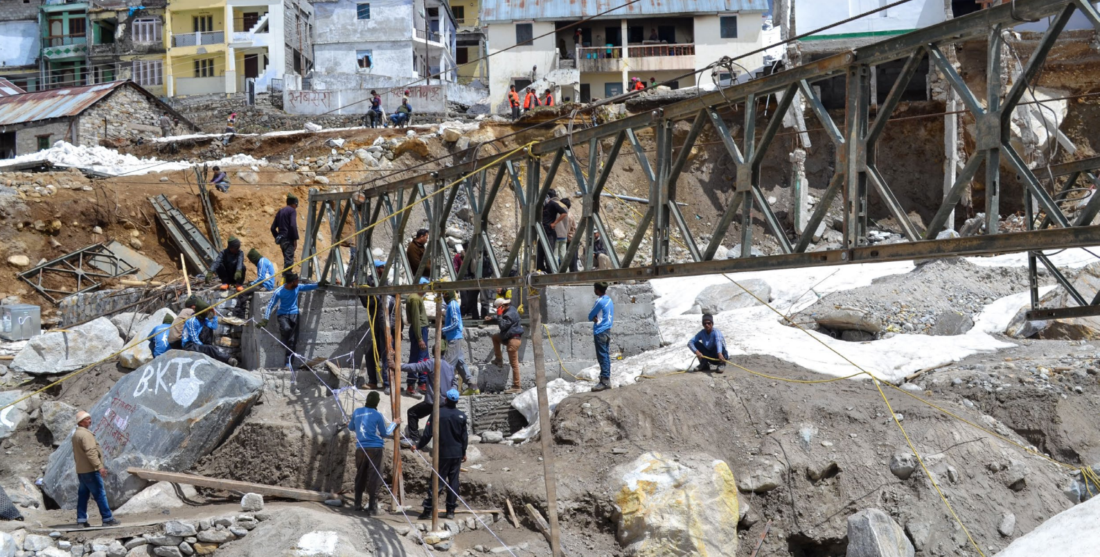
Rebuilding damaged bridges in Kedarnath, India Source: Shutterstock
