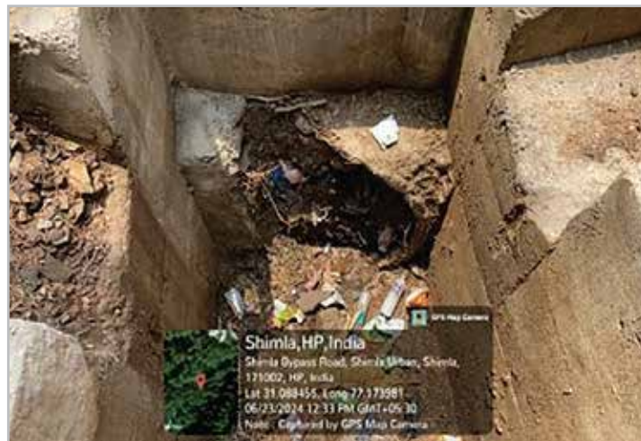
Figure 3: Culvert blockage
