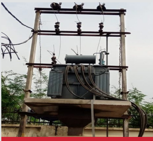
Figure 7.3: Plinth-mounted prefabricated foundation
