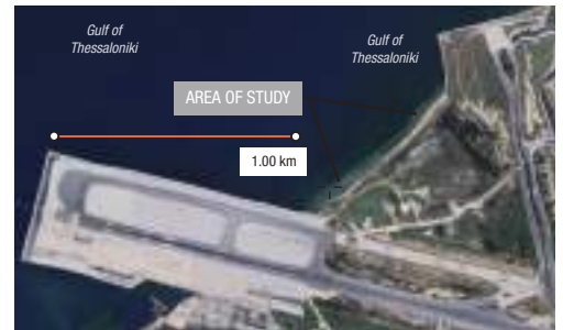
Image 1 – The area of study is located between the two crossing runways (16-34 & 10-28) of Thessaloniki Airport
