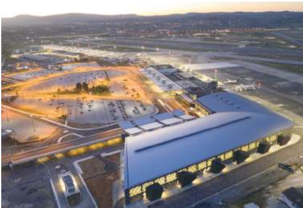
Overview of Thessaloniki Airport
